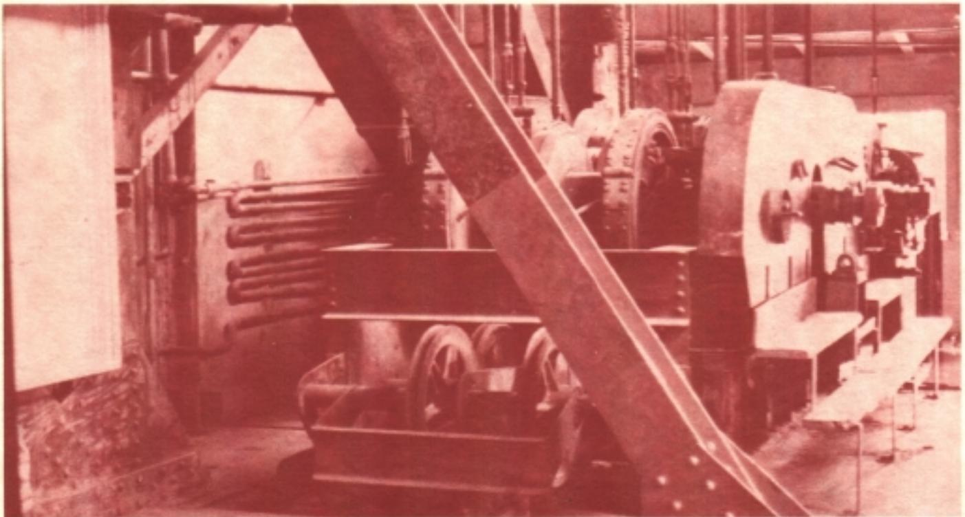
*Hoist machinery connected to winch lines raised and lowered the bucket line or digging ladder.*
