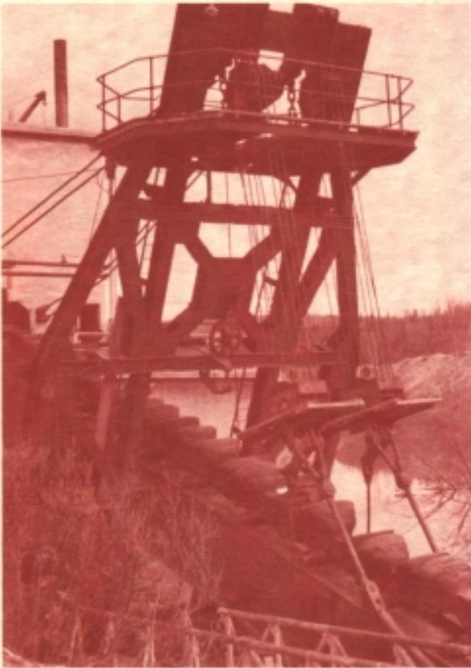
*The bow-gantry lifted the bucket line as it moved gold-bearing gravels into the dump hopper at a rate of 22.2 buckets per minute.*
