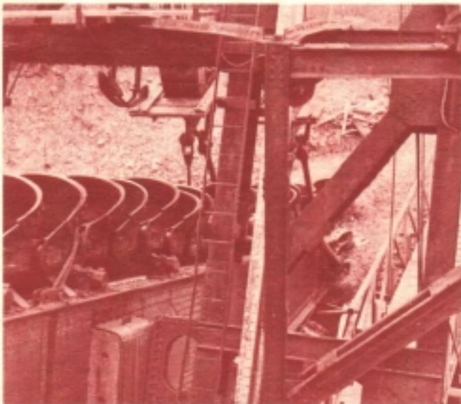
*Manganese steel buckets weighting 1,583 pounds each were mounted on the digging ladder assembly. Each bucket had a capacity of 6 cubic feet.*
