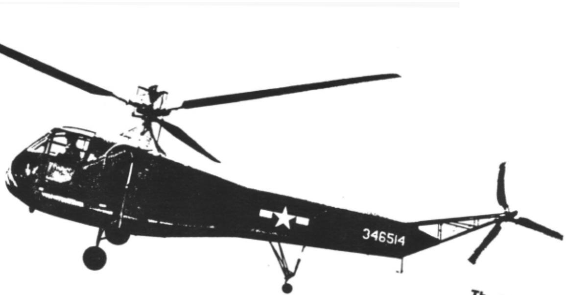
*The Sikorsky R-4 was the world's first mass-produced helicopter. It was based on the VS-300 design. The R-4 was flown by American military forces during WWII, and used on the first successful helicopter rescue to retrieve downed aviators behind enemy lines in Burma.*
