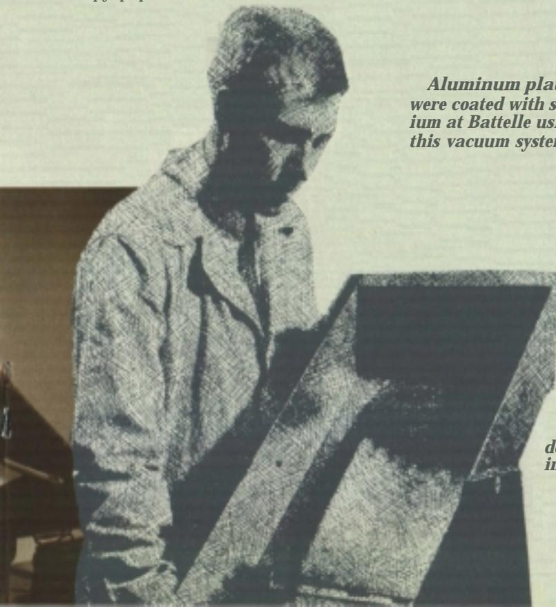
*Aluminum plates were coated with selenium at Battelle using this vacuum system.*
