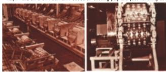
"SKINNER" ROTARY PRESSES. 1930's-early 1950's. Developed by professor Faulds, Clearwater, Fla. and manufactured by Skinner Machinery Co. CLOSE-UP OF "SKINNER" PRESS showing male/female features which pressed pulp and juice from fruit halves.
