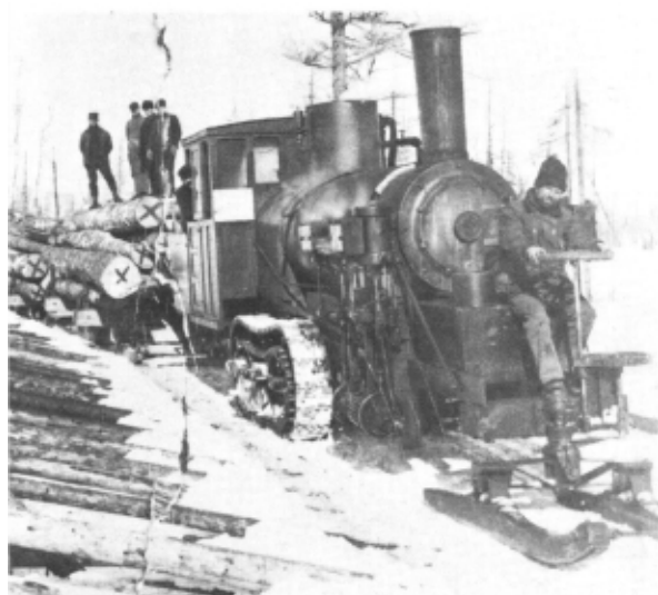
A Peavey Log Hauler, Traction was obtained by revolving screws.
