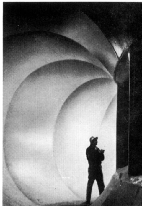
FROM THE 18-FOOT diameter penstock, water will fill the scroll case, surround the stay ring and wicket gates. (FIGURE 5)
