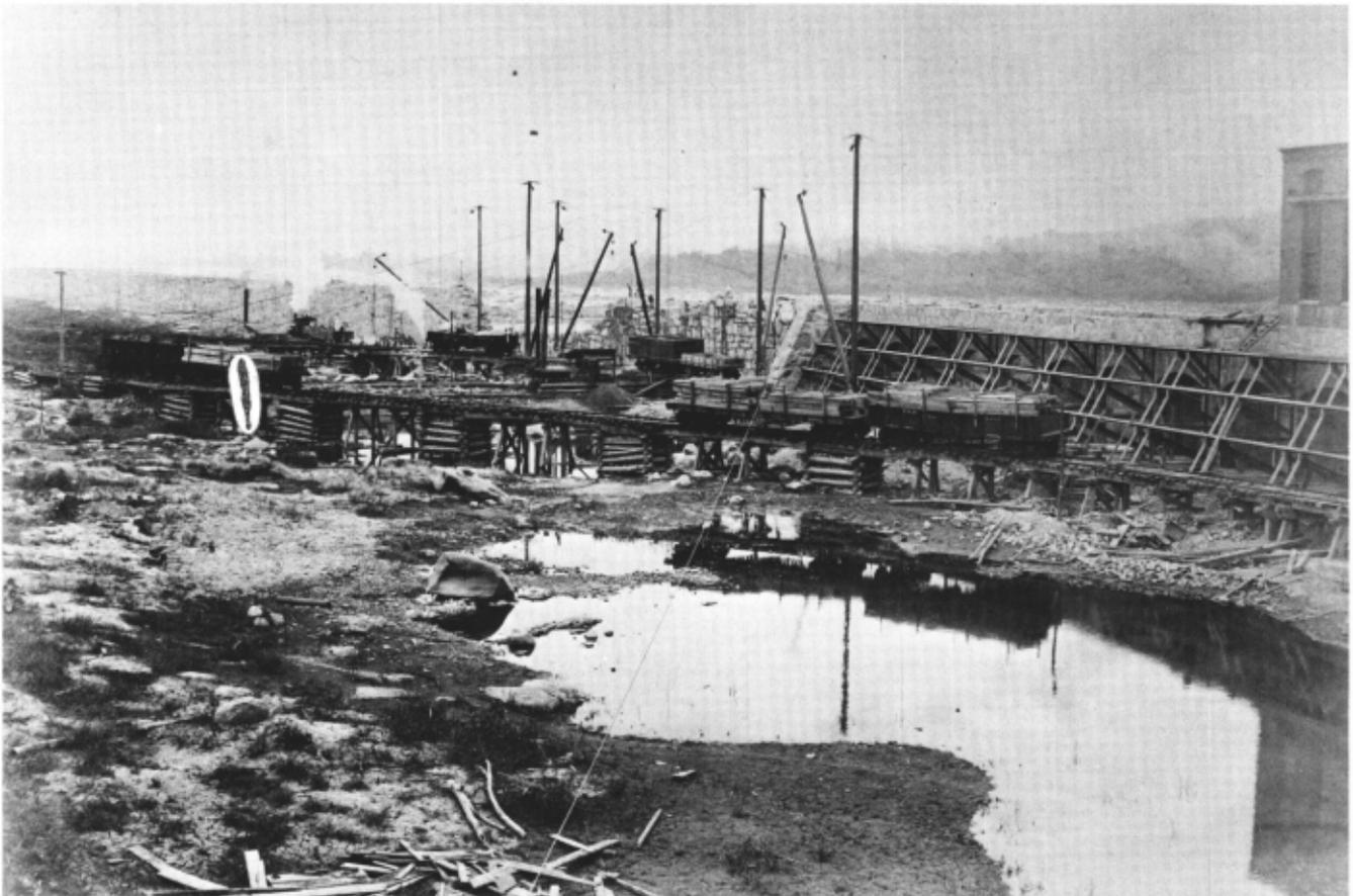
concepts in the making of electricity. The waters of the Susquehanna River are trapped and directed by a 5,000 foot diversion dam and a 3,000 foot headrace. The headrace was designed to complement natural rock formations and river islands existing in the river.
