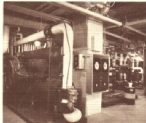
This heat pump, a part of the new installation, has the capacity to run 300 tons of refrigeration. It is one of two heat pumps which heat and cool the Commonwealth Building. When both pumps are running, the system can handle 700 tons of refrigeration.
