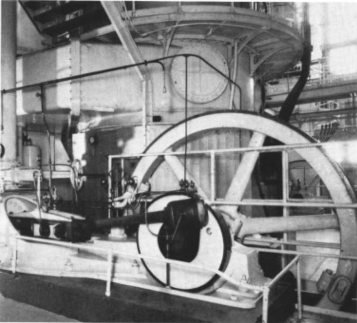
1907 vintage horizontal Tandem Weiss Crank and fly-wheel air pump produces 15 ft. of water vacuum in the barometric steam condenser for each vertical steam turbine.
