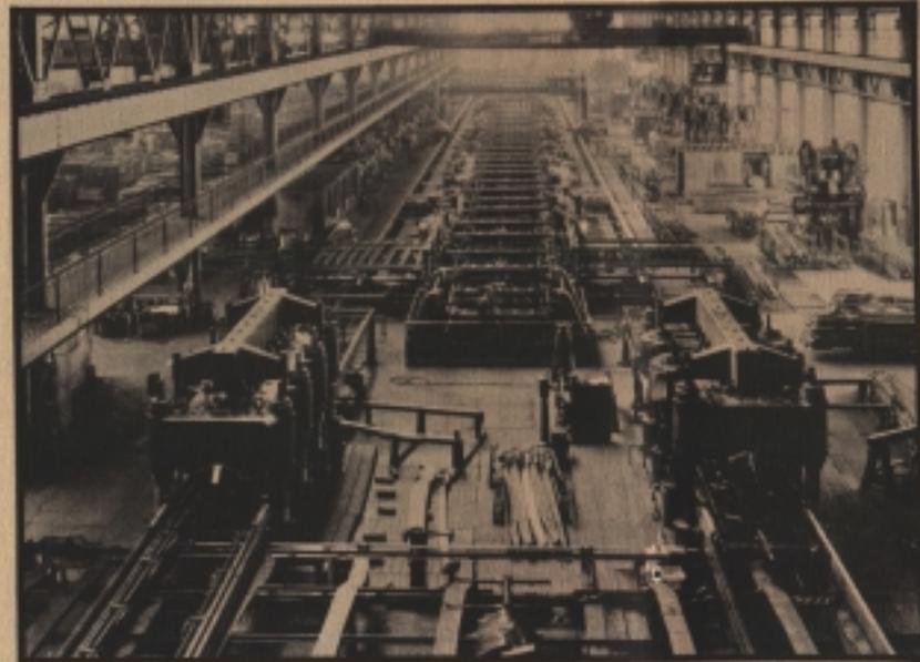
At 19 different stations a number of machining operations were performed along these parallel ways for right and left hand side bar assemblies.
