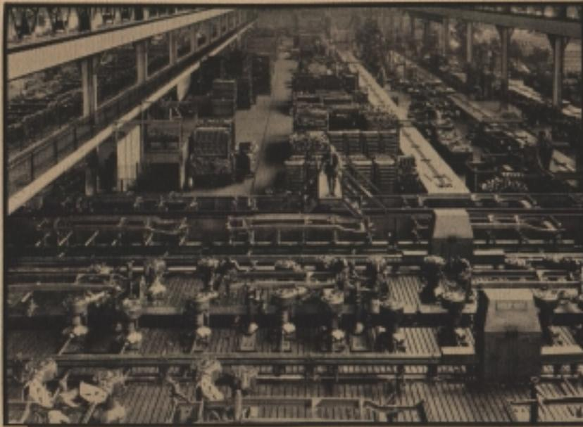
This was a portion of the general assembly unit showing the frames on the truck and the riveting machines closing in to set the rivet heads.
