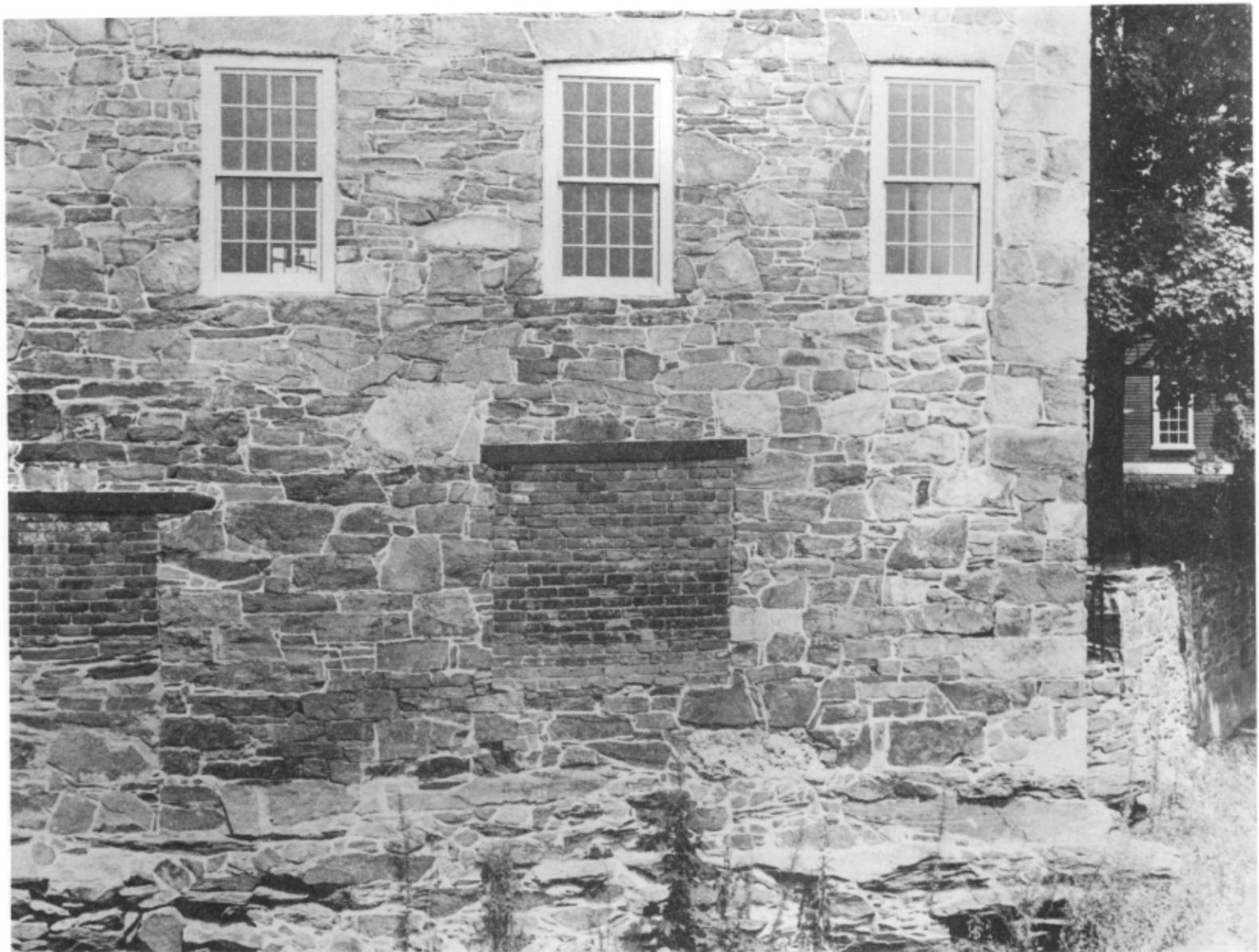
Cast Iron Shafting Used as Lintels
