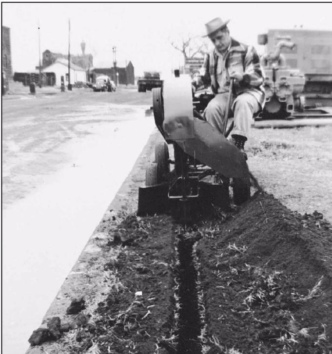
*Ed Malzahn digs a 4-inch wide trench with the DWP trencher. The spoils are piled neatly to the side of the trench.*
