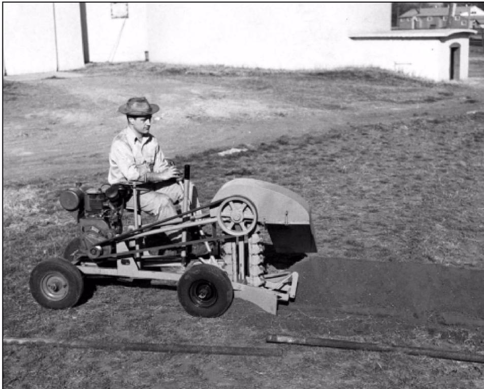
*Ed Malzahn prepares for the installation of a water line. The DWP allowed small diameter pipe to be installed without using manual labor to dig the trench.*
