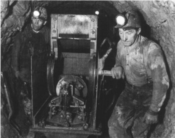
This photograph is seen from the front with the bucket in the discharge position.
