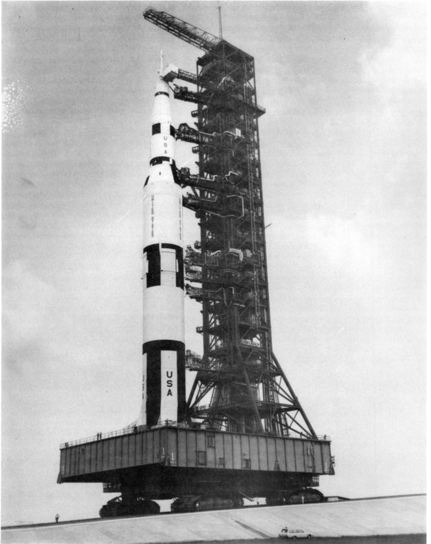
TRANSPORTER WITH MOBILE LAUNCHER & SATURN V
