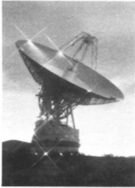
ABOVE: THIS DEEP SPACE NETWORK ANTENNA IN CALIFORNIA'S MOJAVE DESERT, SHOWN IN ITS 64-METER-DIAMETER CONFIGURATION, WAS ENLARGED TO 70 METERS TO SUPPORT THE VOYAGER NEPTUNE ENCOUNTER.
