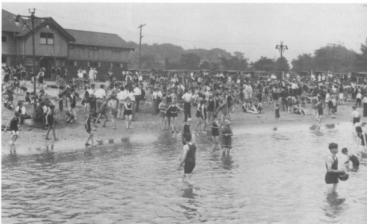
Swimmers enjoyed the expanded shoreline at McKinley Beach, made possible through the excavation of the Milwaukee River Flushing Station tunnel.
