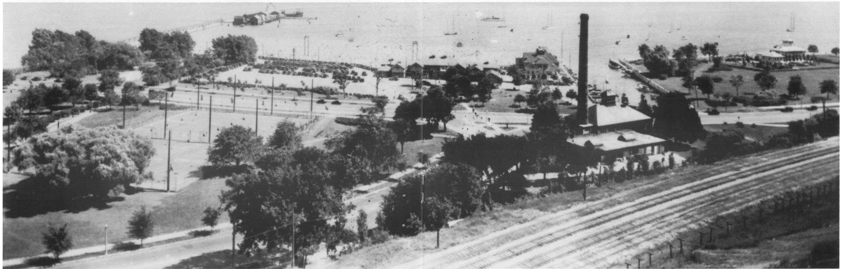
At 126 feet, the flushing station's brick smokestack was a prominent feature along Milwaukee's lakefront for many years. It was removed after the pump's power supply was converted from coal to electricity in 1912.
