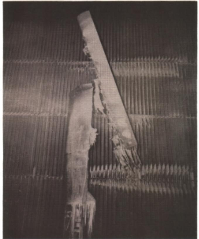
*First icing spray system—a rotating spray bar. Ice formed on the bar from spraying droplets upstream. Spray nozzles produced droplets that were much too large to simulate natural icing.*
