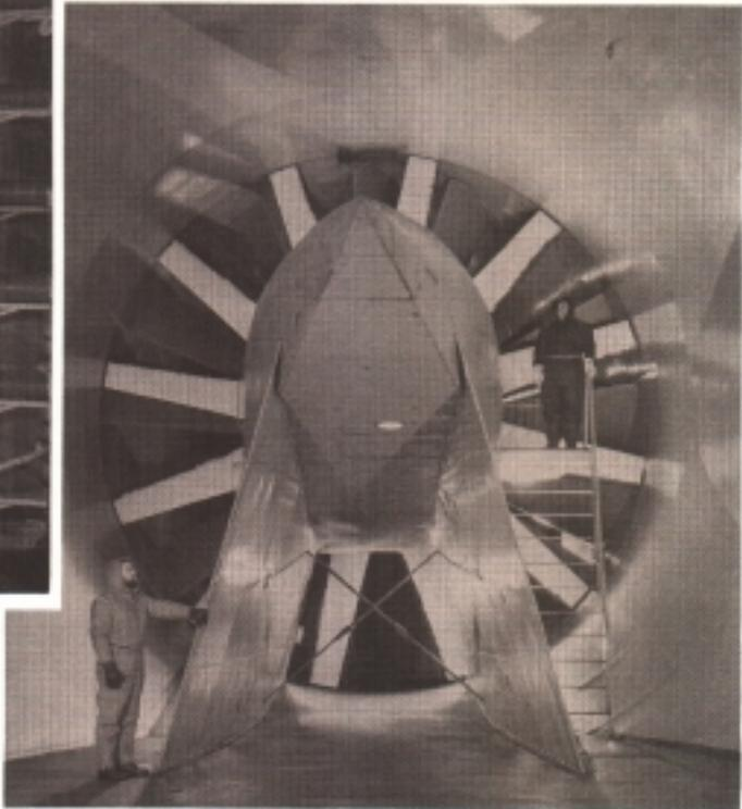
4100-Horsepower drive fan (24-ft diameter) for IRT (looking upwind).
