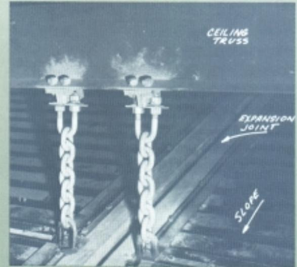
The ceiling deck supports 13 inches of insulation and is hung from the roof trusses. Only the chains go through the insulation. Shown during construction
