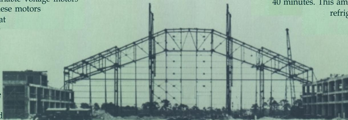
This 1945 photograph shows the concrete side buildings supporting the first roof truss, which is 24-feet thick. The span is 254 feet.
