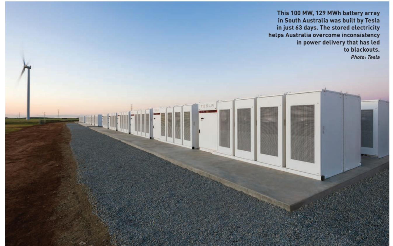
This 100 MW, 129 MWh battery array in South Australia was built by Tesla in just 63 days. The stored electricity helps Australia overcome inconsistency in power delivery that has led to blackouts.
