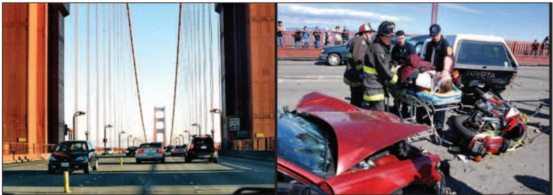
*Lights, paint, and plastic delineation for lane separation lead to head-on, crossover accidents.*
