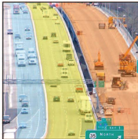
*Moveable barrier provides three lanes into the Twin Cities in the AM, and three lanes back to WI in the PM.*
