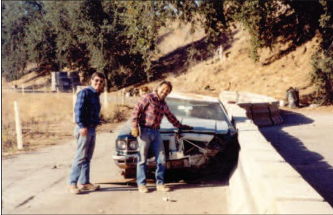
was pulled into a chain of barrier set across the roadway at a given angle. When the vehicle reached the end of the guide wire, the pulling cable would disconnect and the vehicle would freely travel the remaining distance into the barrier. After running twenty to thirty tests, Mr. Nordlen had enough data to submit the results to the Federal Highway Administration and the system was accepted for use on the Federal Highway System.
