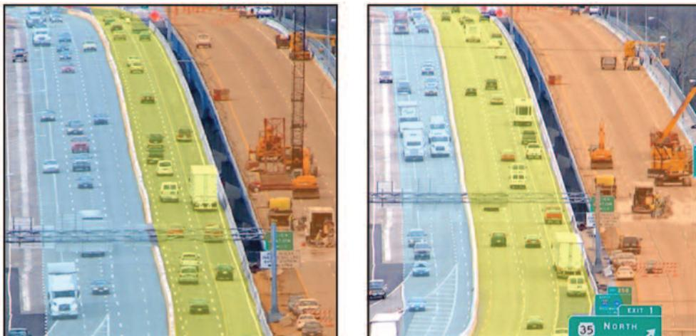
*Moveable barrier provides three lanes into the Twin Cities in the AM, and three lanes back to WI in the PM.*
