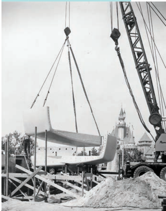
The Monsanto House of the Future was built from plastic wings that were trucked to the site and fused to a concrete base. The idea was that this sort of house could be set up anywhere—and quickly.
