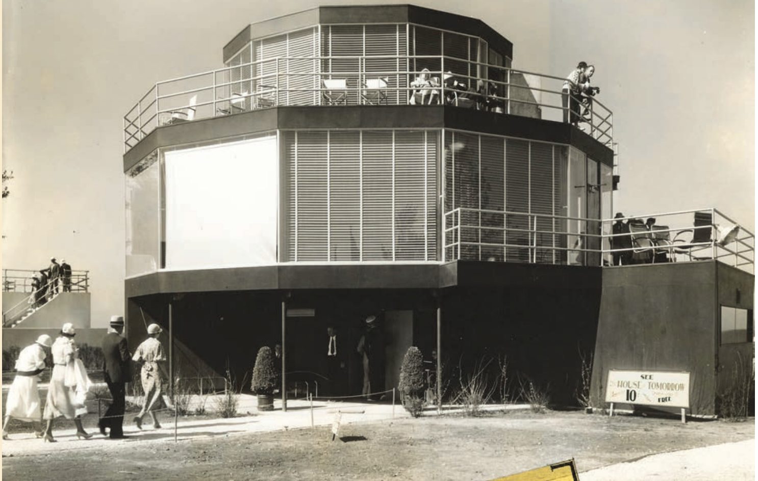
The House of Tomorrow at the Chicago Century of Progress Exhibition hinted at a future where airplanes would be common. The circular plan led to some odd-shape rooms, however, and the floor-to-ceiling windows led to overheating.
