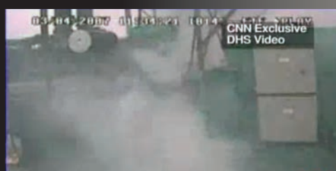
Stills from a video of the Aurora Generator Test, a simulated attack by hackers against a 2.25 MW generator that was connected to a substation: (Top) The generator gets out of sync and starts to bounce; (Middle) bits start flying off the generator; (Bottom) black smoke envelops the machine as the generator is destroyed.
