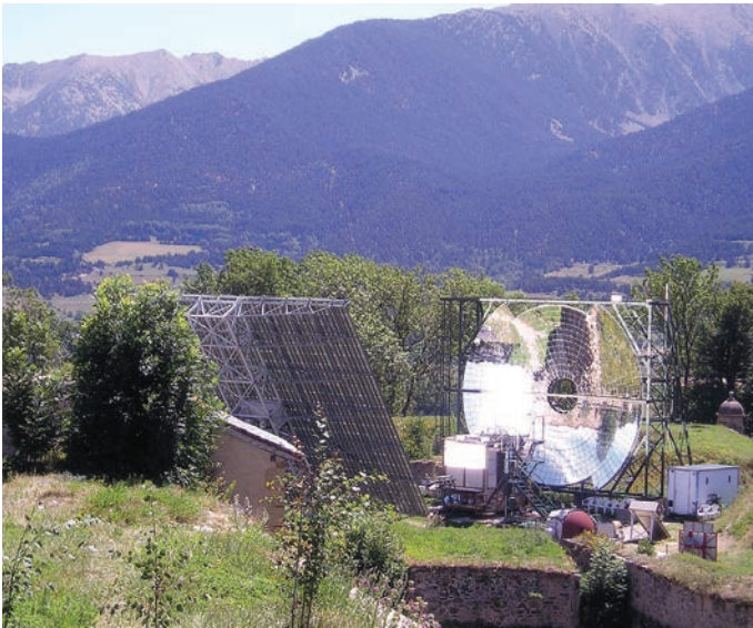
Facilities such as the Mont-Louis Solar Furnace (above) and the Odeillo Solar Furnace (right and on the opening pages) concentrate sunlight to conduct thermochemical experiments.
