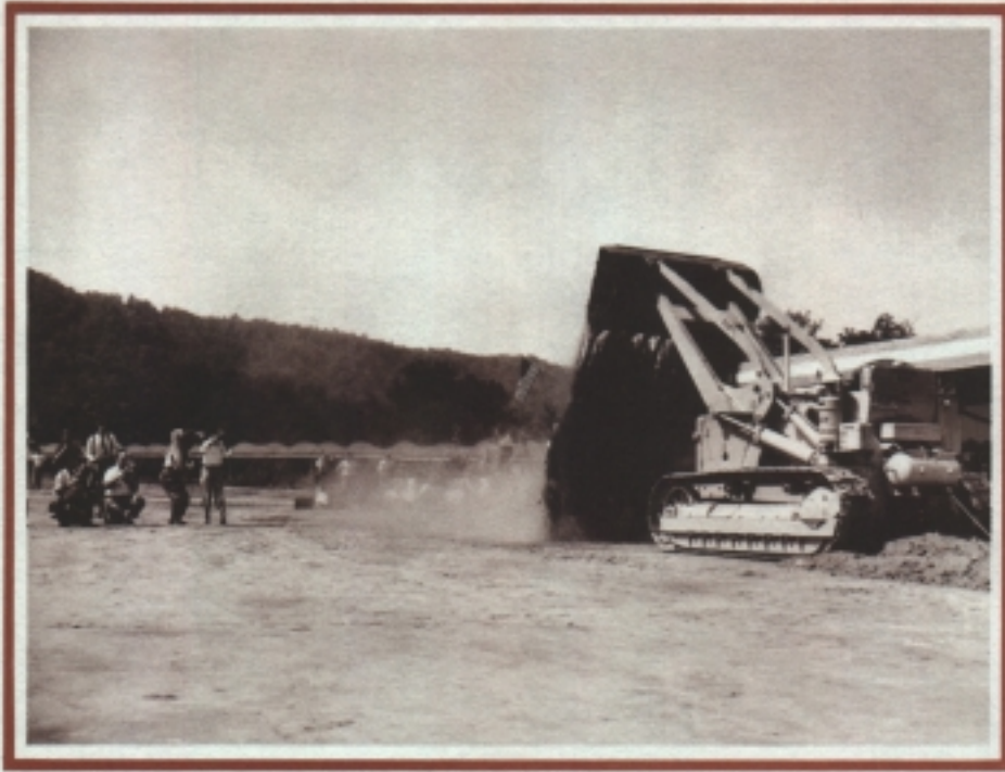
GROUNDBREAKING CEREMONIES featured a large highlift which when electronically activated by President Eisenhower over 1,200 miles away, turned the first scoop of ground for the Shippingport project. When this occurred, the crowd at the ceremonies, sensing the historic significance of the moment, rose to its feet and applauded. Pictures of this occasion were featured worldwide by newspapers, television and movies.
