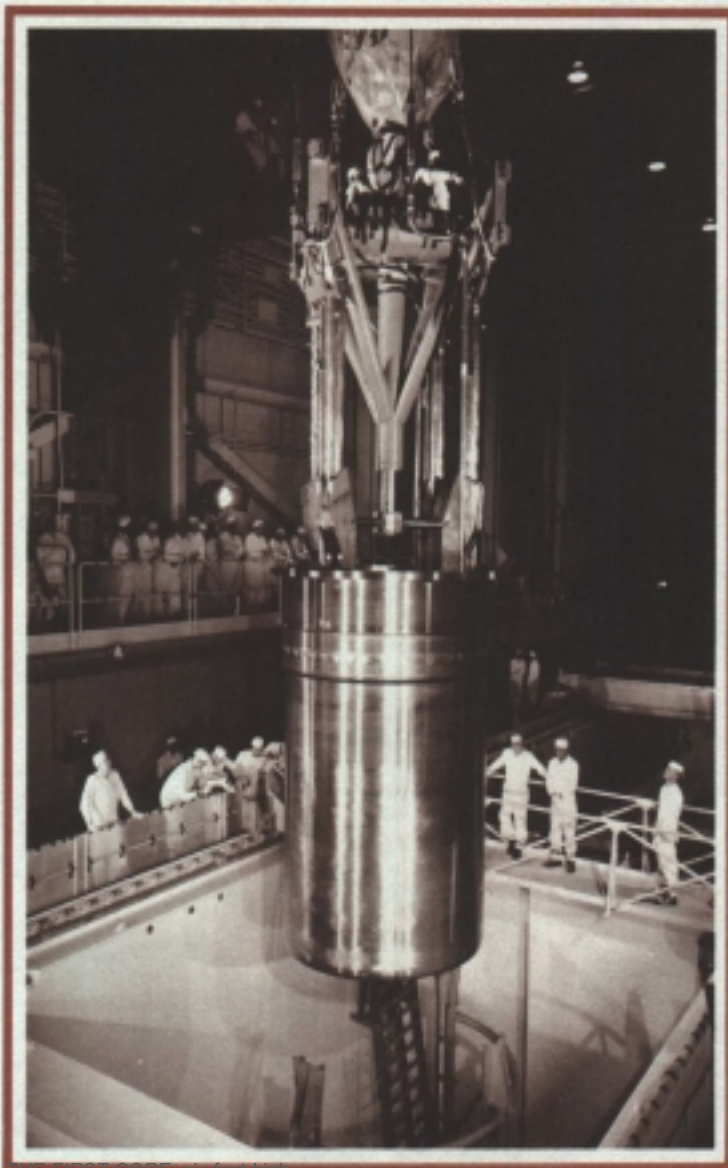
THE FIRST CORE, six feet high and seven feet in diameter, weighing 58 tons and containing 14 tons of natural uranium and 165 pounds of high-enriched uranium, was installed in October, 1957. It took more than eight hours to lower the core, the heart of the reactor system, into position with only six-hundredths of an inch clearance between it and the walls of the steel container known as the pressure vessel.
