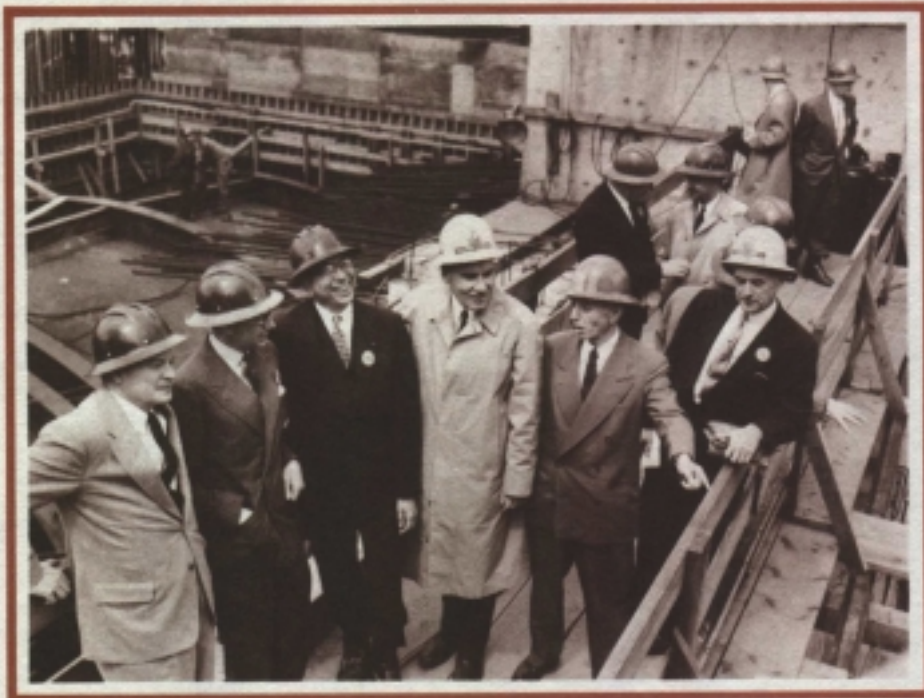
NUCLEAR TECHNOLOGY AND DIPLOMACY mixed together during a tour of the Shippingport construction site by representatives of Great Britain. Participating in the tour were from left, Charles H. Weaver, Vice President, Westinghouse Electric Corporation, Sir Edwin Plowden, Chairman of the United Kingdom Atomic Energy Authority, Lewis L. Strauss, Chairman of the AEC, Philip A. Fleger, Chairman of the Board, Duquesne Light Company, Admiral H. C. Rickover, Chief of the Naval Reactors branch of the AEC, and H. Briggs, Jr., Duquesne's Manager of Advertising and Public Relations.
