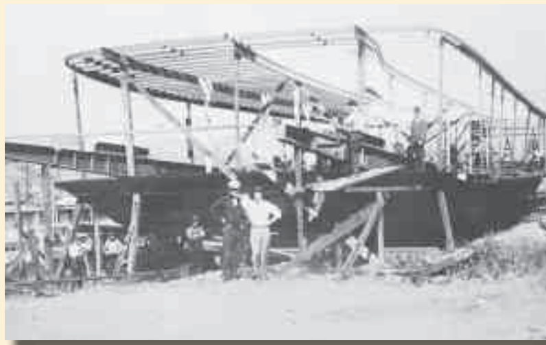
Construction on the Idlewild.
