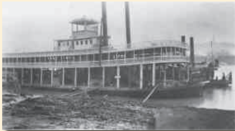
Idlewild during construction at Rees yard.
