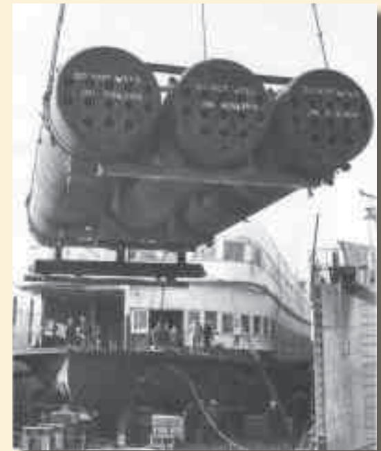
Lowering new boilers into position on the Belle of Louisville.
