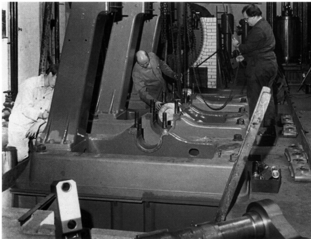
No steam restoration task is too big or too small for Kew's full time staff and volunteers who are pictured erecting the 'Triple' in the Museum's steam hall.
