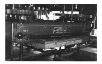
A three speed drive has been incorporated in the design of the press to insure that as much juice as possible is squeezed from the apples. According to their catalog, "This (the three speed drive) enables the operator to run down until the head strikes the cheese; then shift to the medium motion, until the bulk of the cider is extracted, and to finish on the slow speed, the power [force] increasing as the speed decreases."
