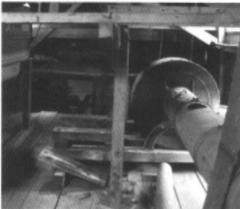
Belt driven fan for Munger's pneumatic system of cotton ginning.
