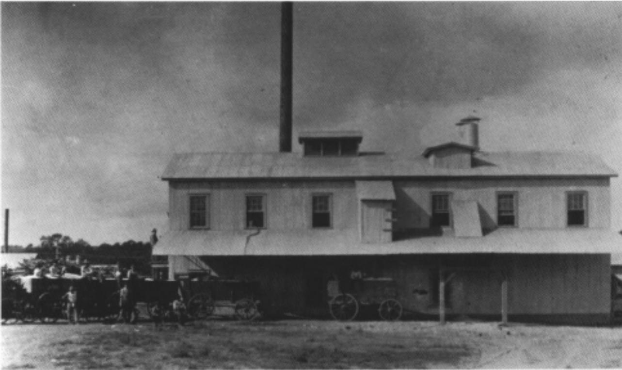
Photograph of the Burton Farmers Gin as originally constructed. Notice the steam boiler smoke stack rising above a simple roof line. In 1925, a seed house was added to the front of the gin and the roof line altered to house seed elevators and stick removal equipment. An engine room with a business office above it was added to the left side of the building to house the Bessemer Type IV oil engine.
