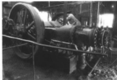
Bessemer engine drives the line shaft through a clutch on the right with the clutch handle shown in the foreground.
