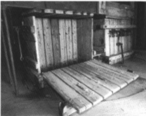
Double box bale press allowed cotton to fill the box on the right while pressing and unloading a bale of cotton from the other box.
