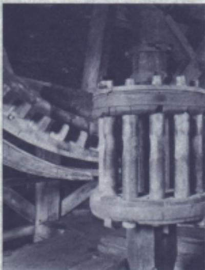
*The lantern wheel and main drive gear are parts of the grinding mechanism visible on the third floor.*
