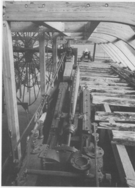
Wood and iron pitman arms on each side of the Cairo served as connecting rods between steamdriven engines and paddle shaft cranks.
