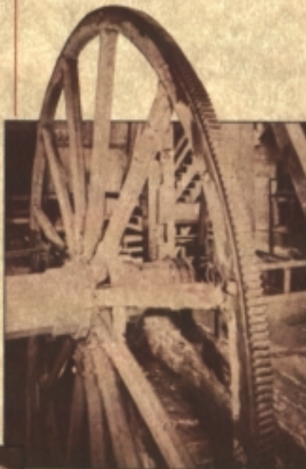
The large gear wheel which ran the blowing tubs and provided the cold air blast measures 76 feet in circumference.
