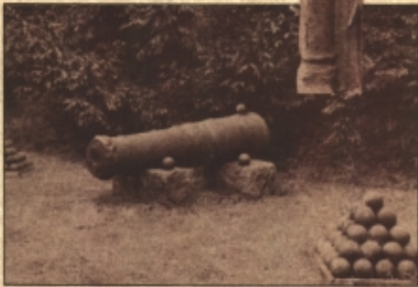
▲ Most iron furnaces were called on during the American Revolution to cast cannon, and Cornwall was no exception. Forty-two naval cannon were cast here, along with much ammunition. This cannon, once displayed on the lawn at the ironmaster's estate, has been returned to the Cast House where it was made, probably in 1775.
