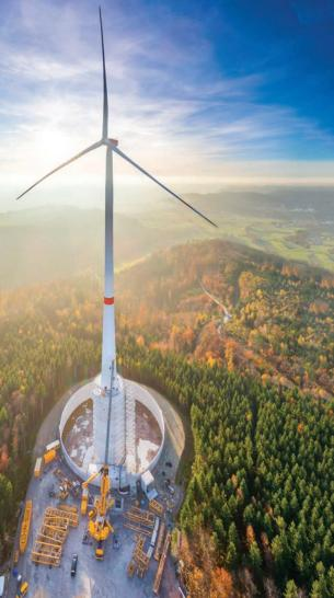
By combining a wind turbine with pumped hydro, Max Bögl Wind AG created renewable energy storage that's more durable than batteries.
