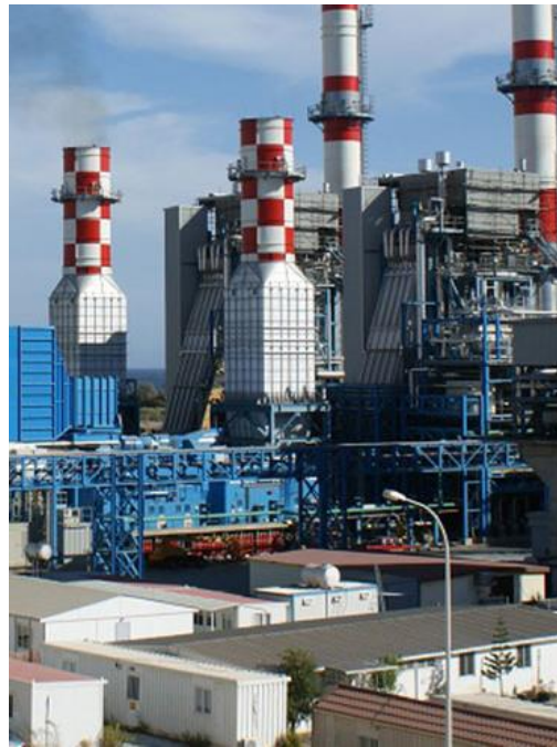
Industrial power generation
