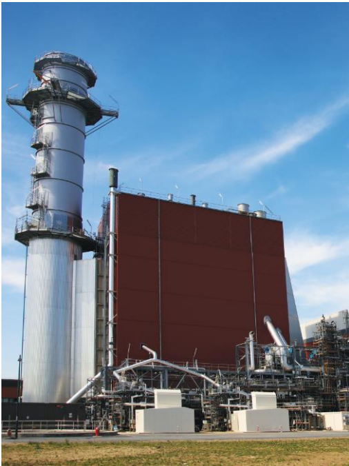
Utility and IPP power generation
