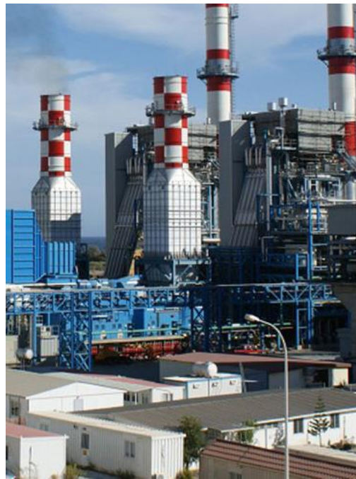
Industrial power generation
