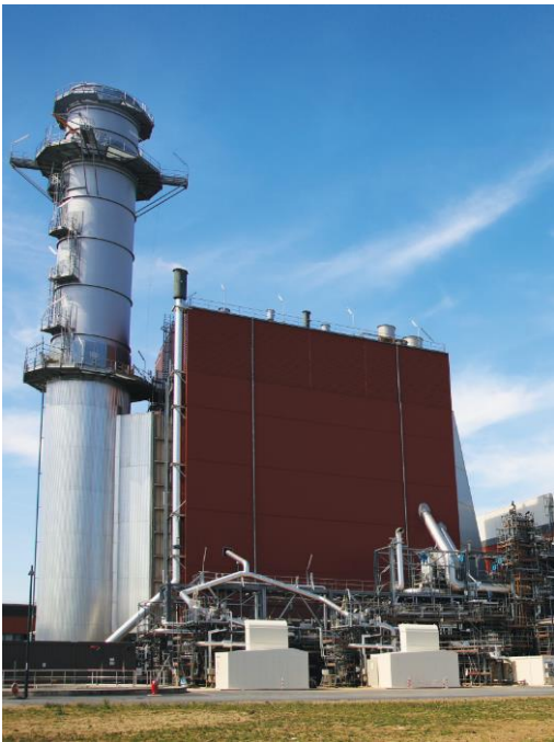
Utility and IPP power generation
