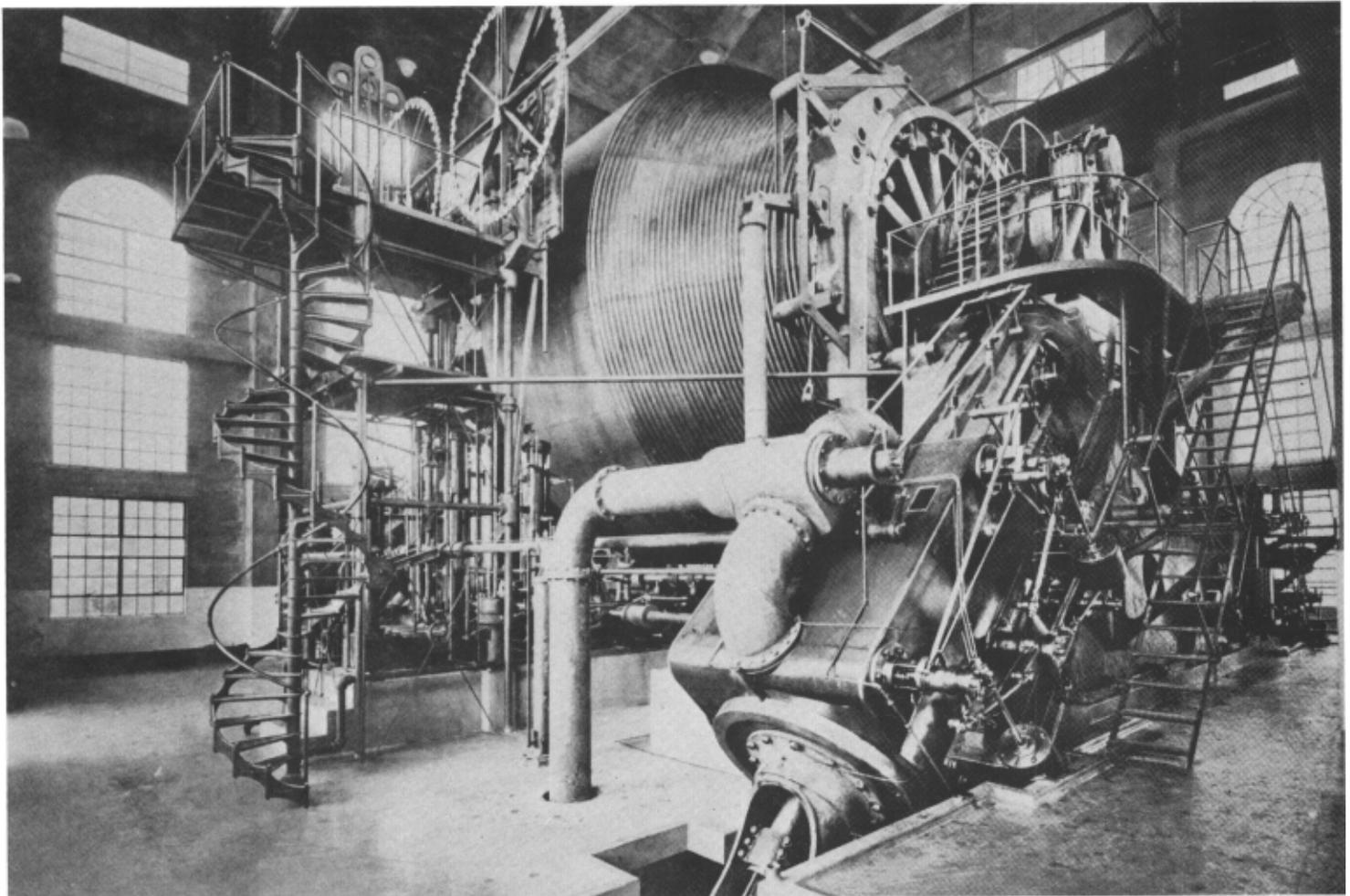
The combined weight of the hoisting engine and the condensing equipment is 1,765,000 lbs.
