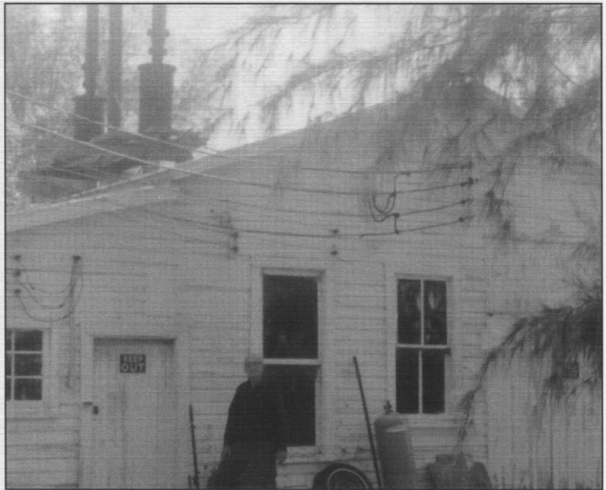
Original Useppa power house with exhaust stacks in Background (1976). Also shown is Useppa Island Chief Engineer, 1923-1924.
