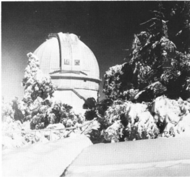
The completed facility.
