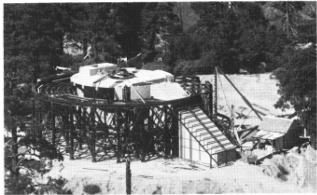
Grinding the rails for the moving dome.
