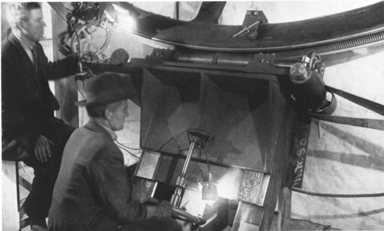
Gashing of one of the 1440 teeth in the 18-foot diameter gear.
