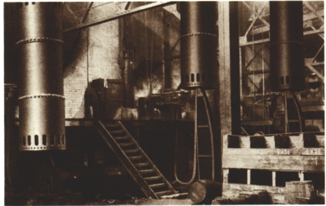
Rivets in these pre- 1930 boiler drums were driven by hydraulic pressure.
