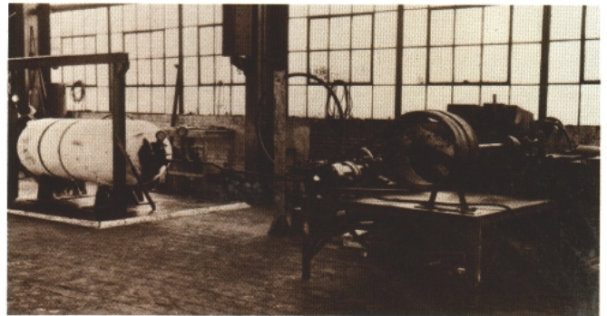
This historic recording shows C-E's first all welded boiler drum in the shop where it was tested to destruction.
