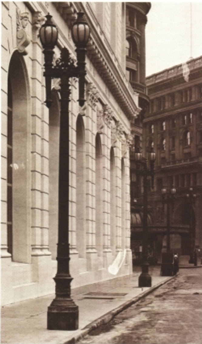
Street Lamps Built by Hendy, 1921
