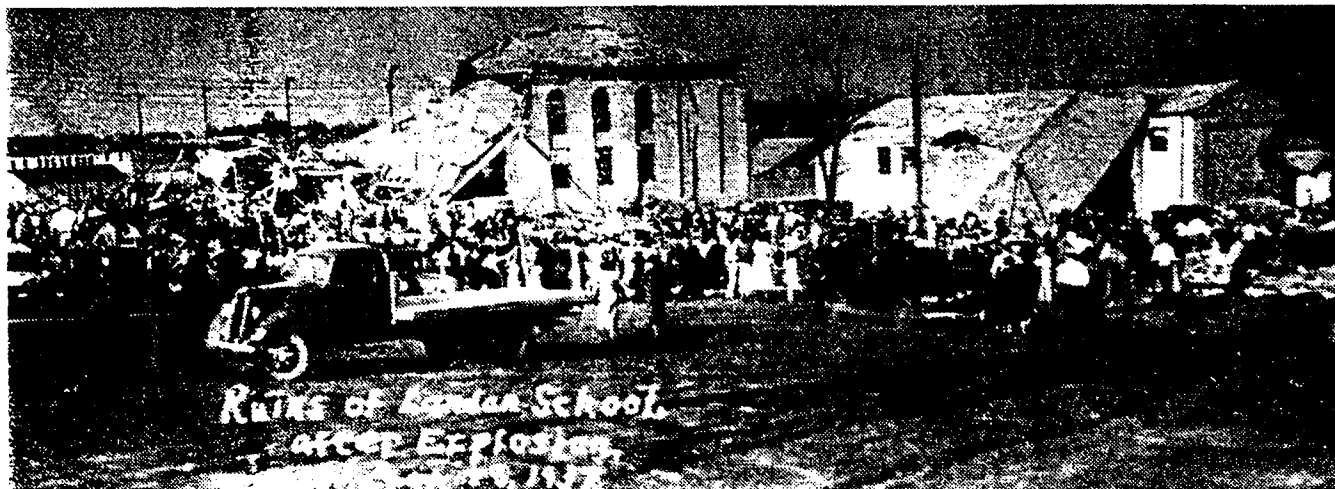
The New London school, viewed from the same spot, after the explosion, which was caused by natural gas.
