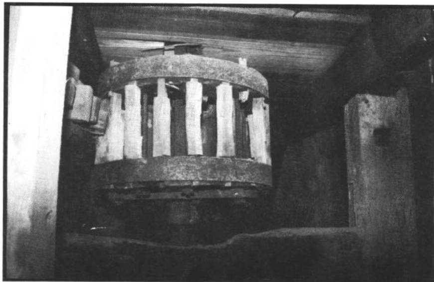
Grindstone Driving Shaft
