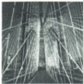
The Brooklyn Bridge. Showing the use of wire rope.
